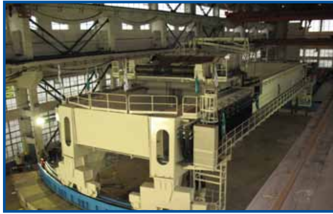
350 ton X-SAM® polar crane (700 ton construction capacity) built in 2008
